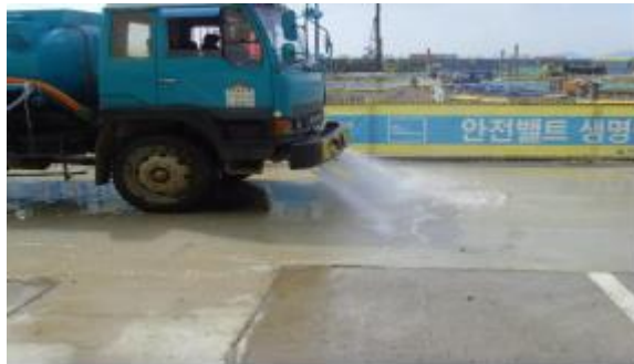
[Water spraying truck]
