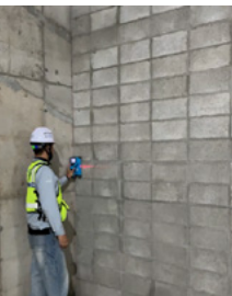
Reinforcement bar detector inspection
