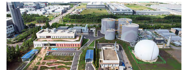
Siheung Clean Energy Center
