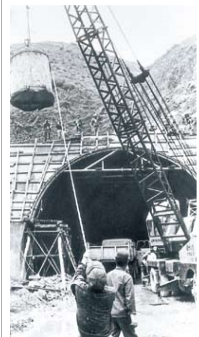
Gyeongbu Expressway project (Dang-jae Tunnel)
